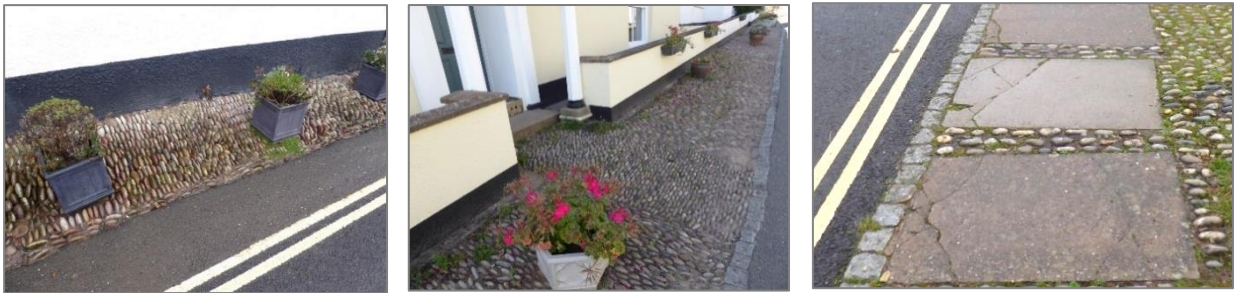
Photos (above): Examples of hard surfaces, showing how original cobbles and granite setts have maintained a better condition than the replacement concrete surface
