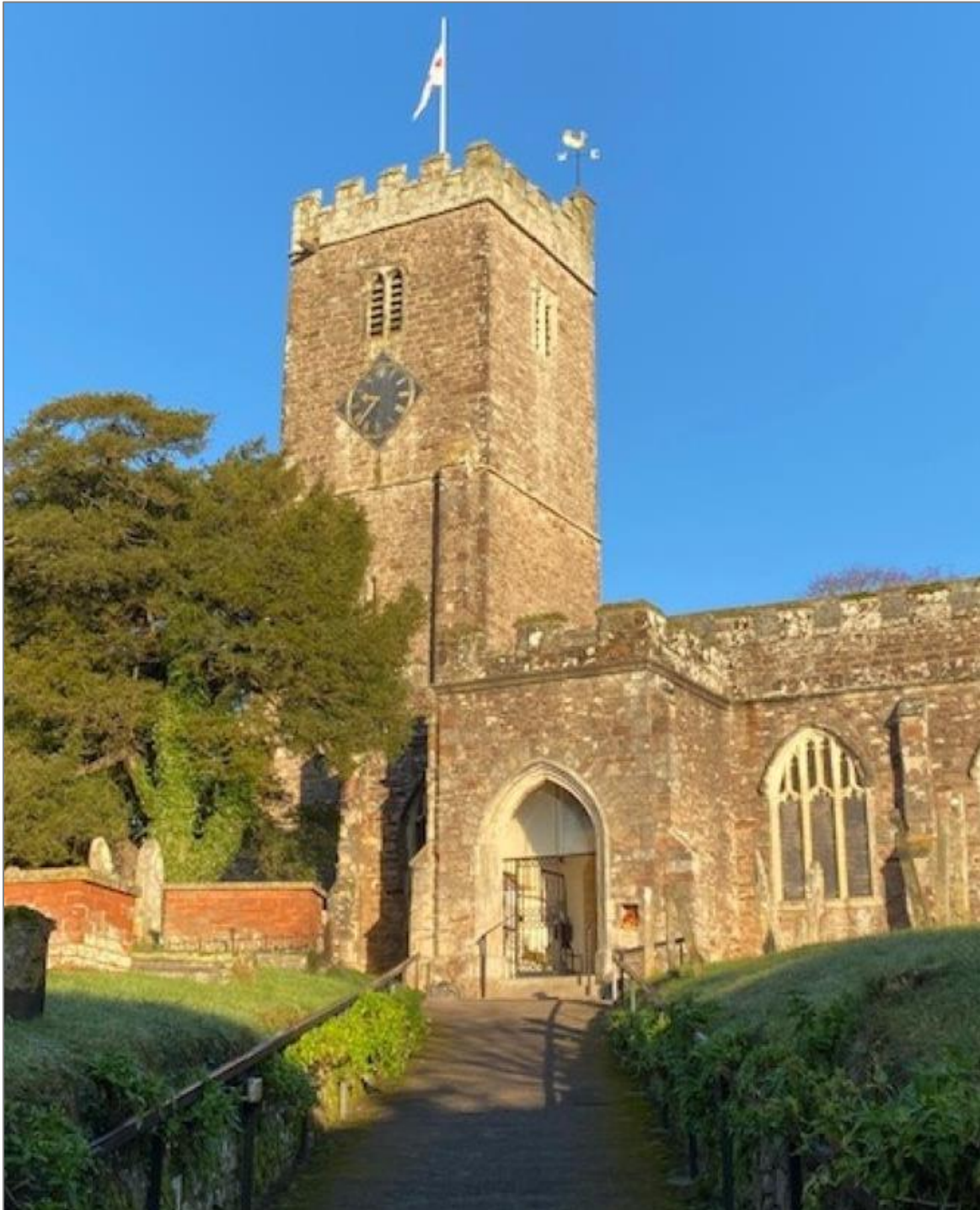
Photo: All Saints Church (Grade 1 Listed), High Street
