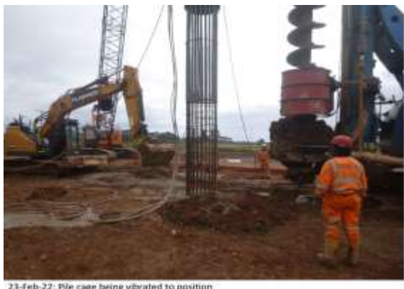
23-Feb-22: Pile cage being vibrated to position
