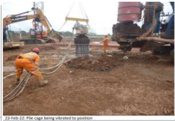
23-Feb-22: Pile cage being vibrated to position
